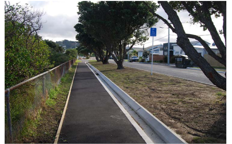
Recently completed berm upgrade with existing boundary treatment
