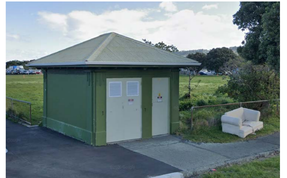
Existing electrical station with mature street within berm
