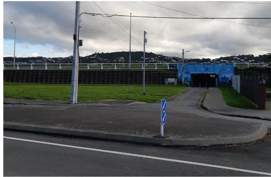
Pedestrian tunnel under Airport runway connecting Miro Street with Rongotai
