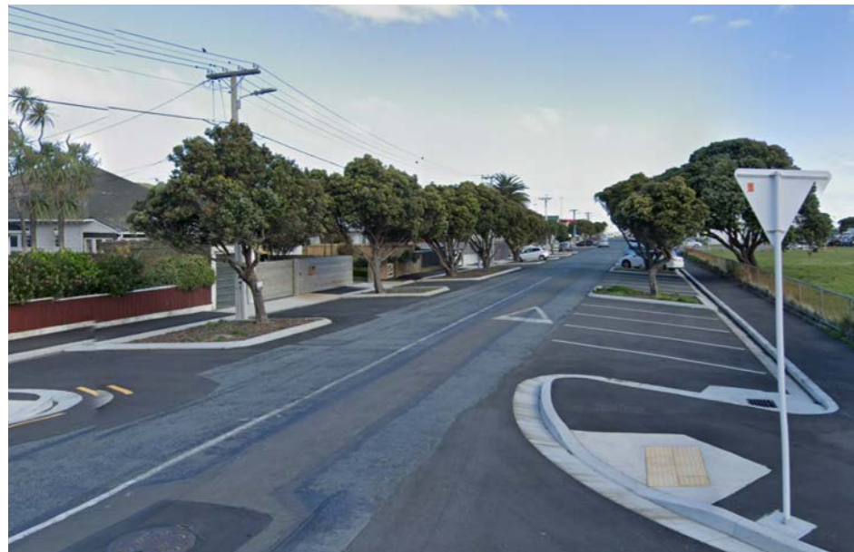
Recently completed street upgrade
