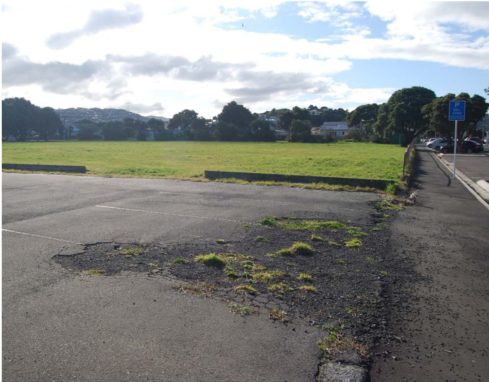
Former carparking area adjacent Kauri Street
