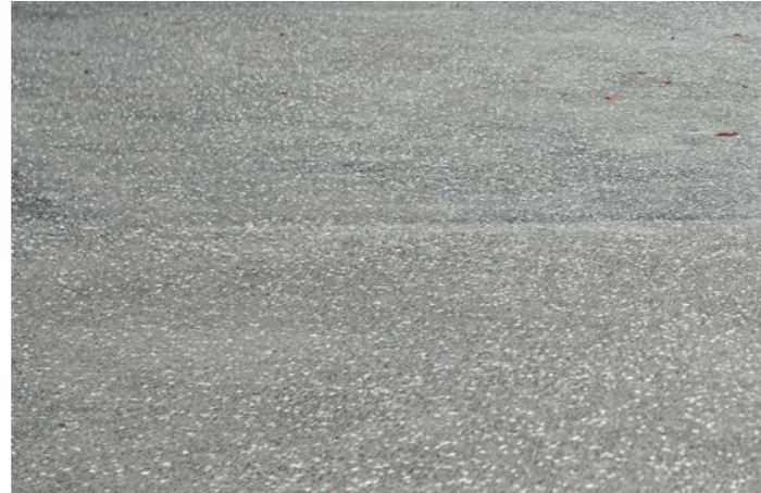
Concrete used for pathways or hardstand. Potential use of a shell mix to reflect coastal area.
