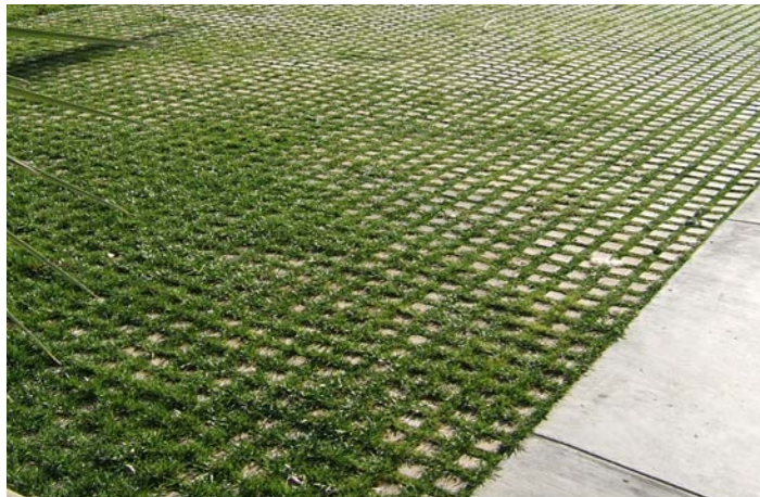
Permeable paving or gobi blocks could be used in parking areas to decrease water runoff. Not suitable for heavy loading vehicles
